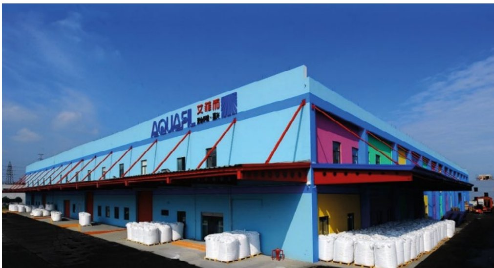
Figure 17 - Visual impact of the Chinese JIAXING plant
