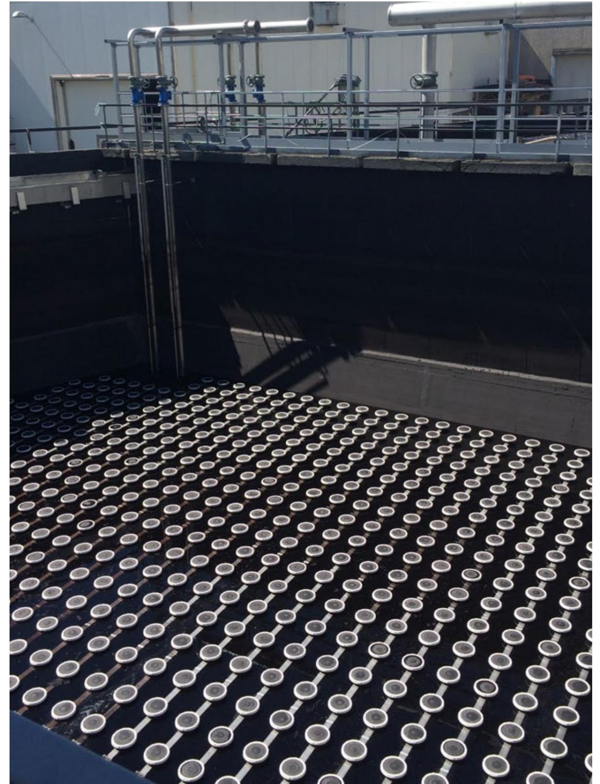
Upgrading of oxidation tank for biological wastewater treatment, installed at Aquaspace (Rovereto, Italy)
